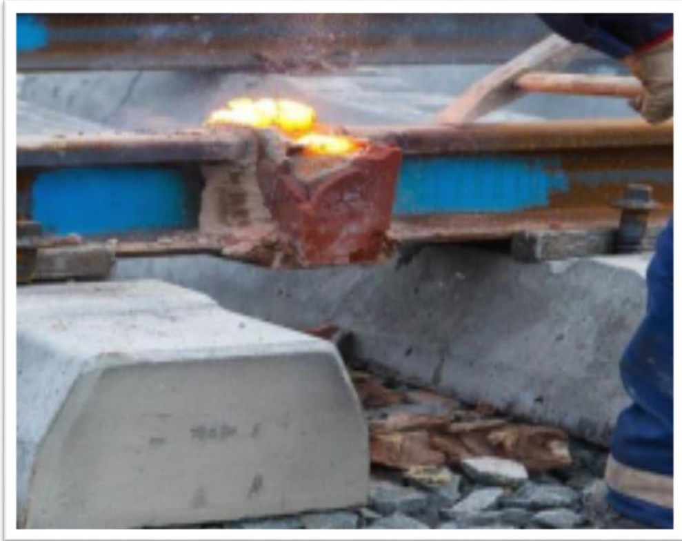
Figure VII.10 : Tranchage du rail
