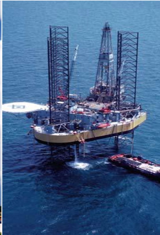
figure 19: offshore rotary drilling
