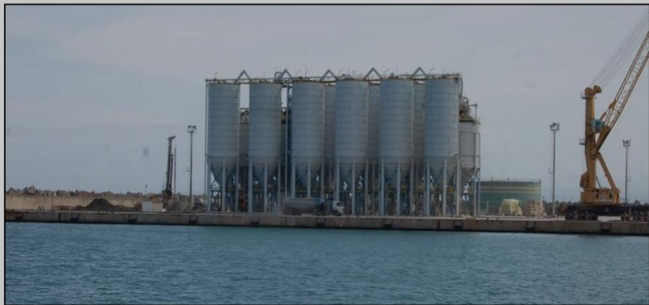
TERMINAL A CIMENT
