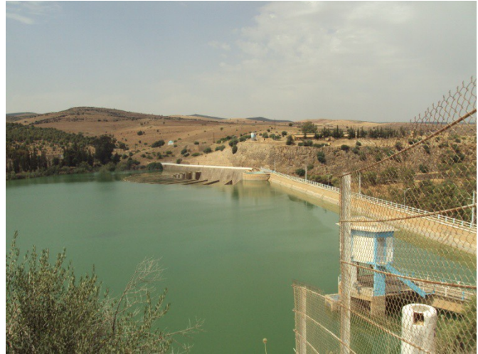
Figure 22 : S14 M.Sfa Barrage Benkhadda (cliché Senouci H, 2015)
