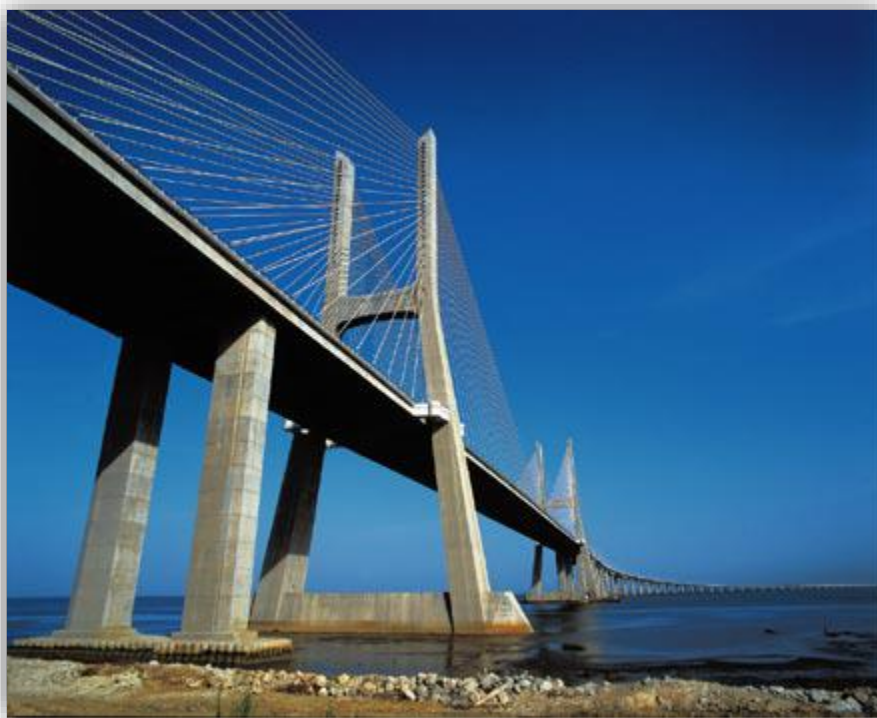
Figure I .15 Pont en BHP [35]
