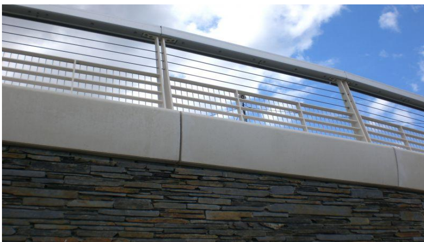
FigureVIII.6 : corniche en béton armé (bord en blanc).
