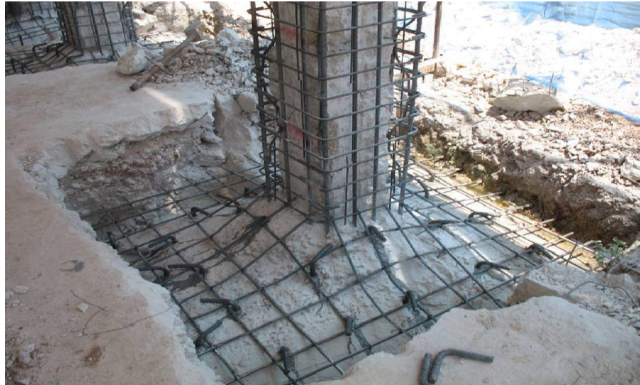
Figure II. 12 : Renforcement des fondations.
