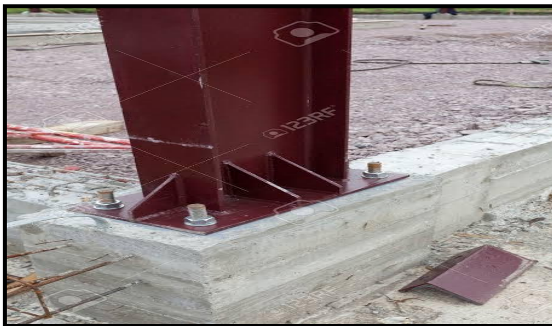
Figure I.13: Poteau en acier
