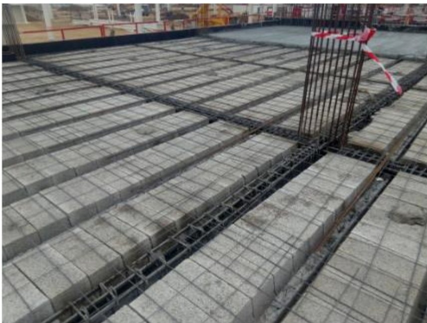
Figure III.1: plancher corps creux.
