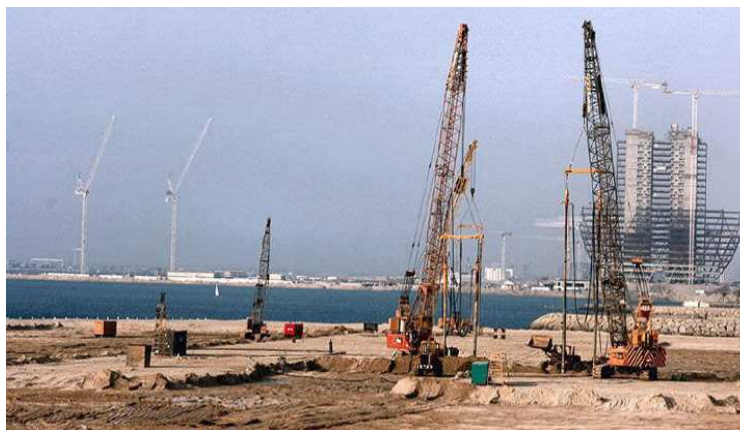
Figure 2.6: Vibrocompactage
