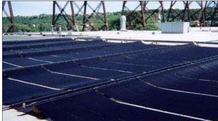
FIGURE III.7: a flat-plate solar collector (unglazed) [5].
