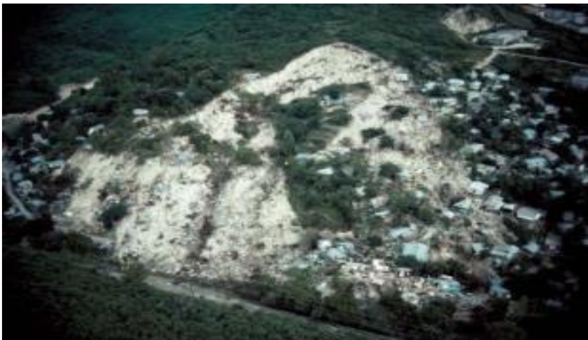
Figure I.6 Glissement de Puerto Rico, 1985
