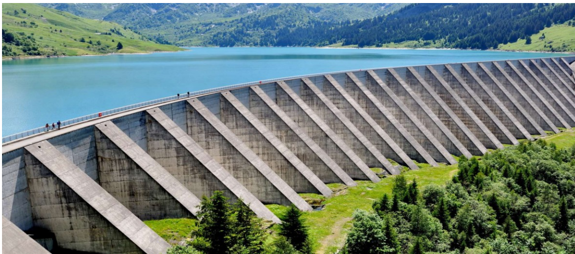
Figure I.13 : Barrage a contrefort
