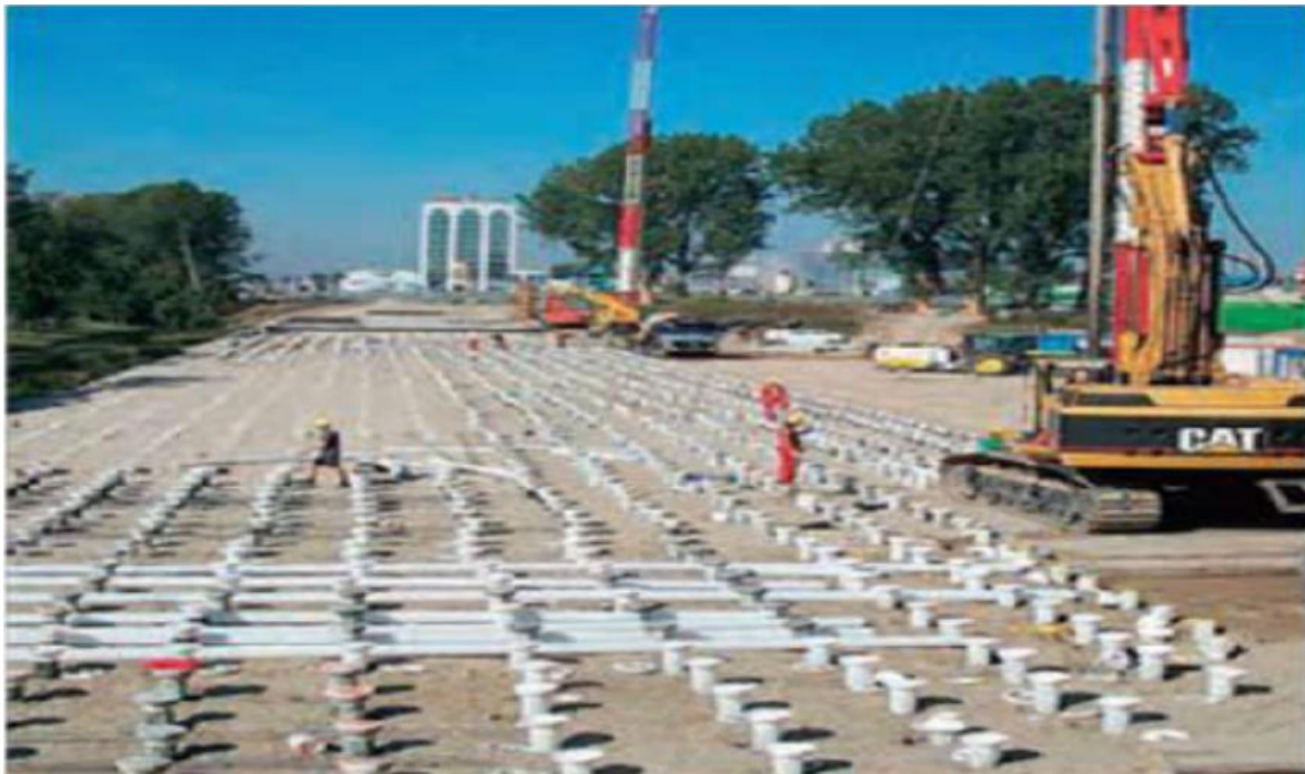
Figure 2.4: Installation des drains.
