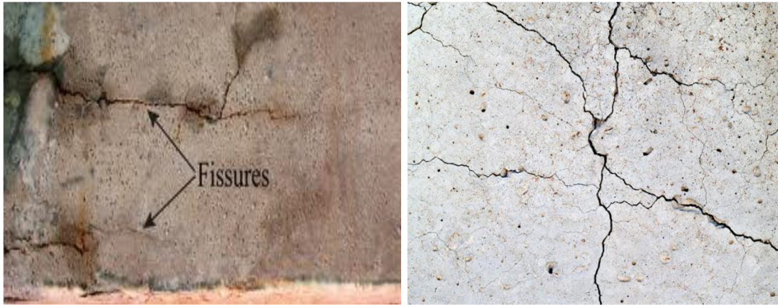
Figure I.1 : Fissuration.
