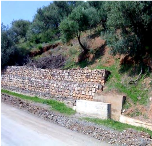
Figure IV.12 :Ouvrage souple, en gabion Sidi Younes Ouzellaguene, Bejaia.
