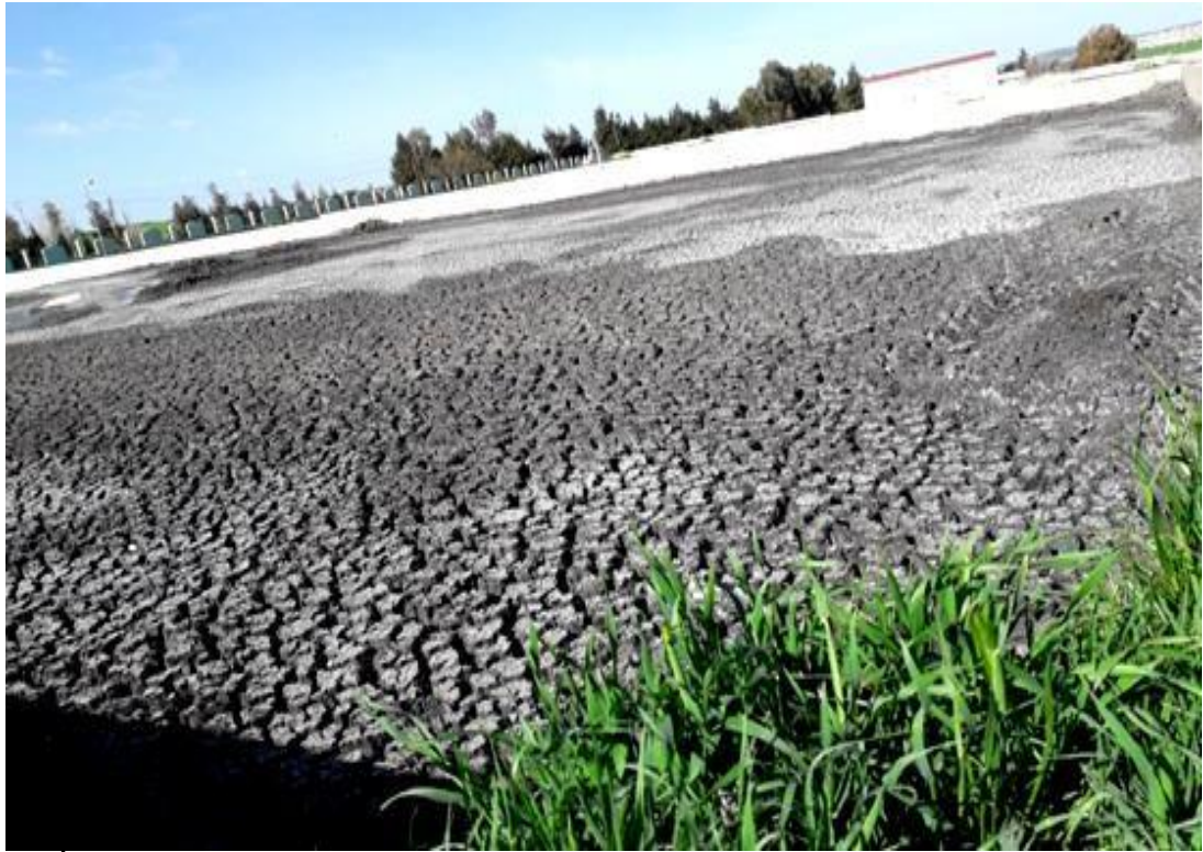
figure III.16: Lits de séchages
