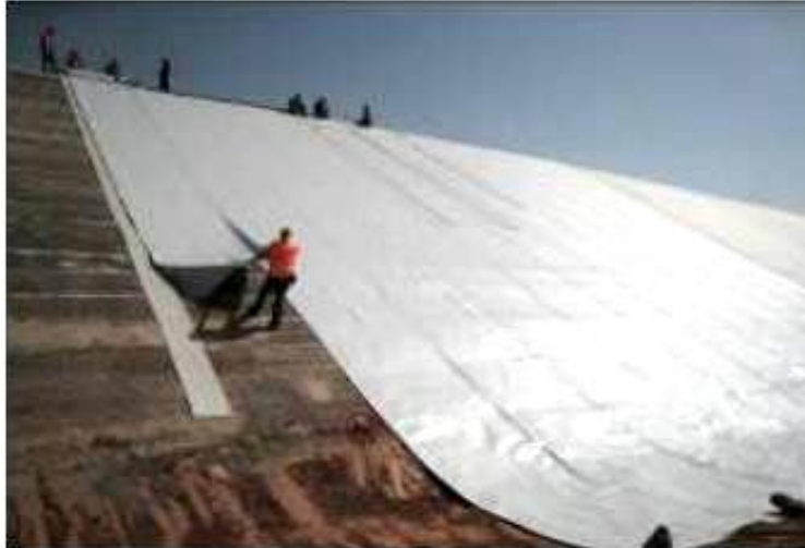
Figure I.5: Pose de géomembrane (Barrage de Sar Cheshmeh, Iran)
