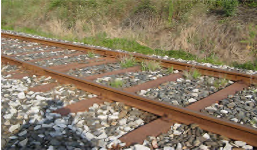
Figure VII.9: Traverse métallique
