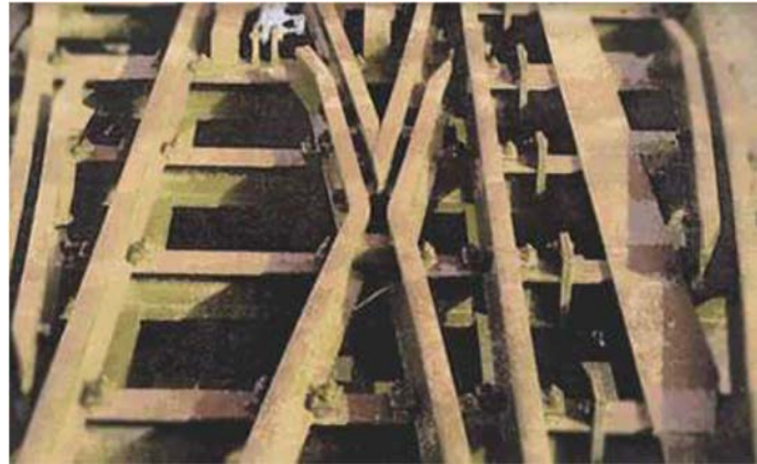
Figure.VIII.N°07. aiguillage
