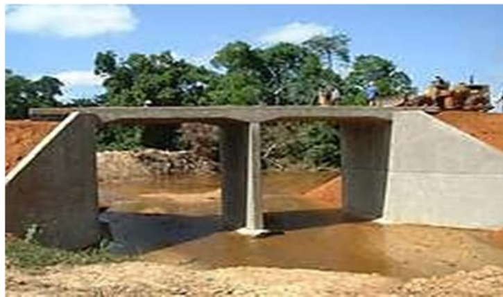
Figure X.N°02: schéma de Dalots.
