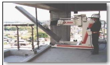
Figure (I.22) : Robot de construction
