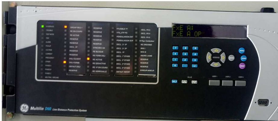
Fig V.4. Protection de distance (General electric D60)
