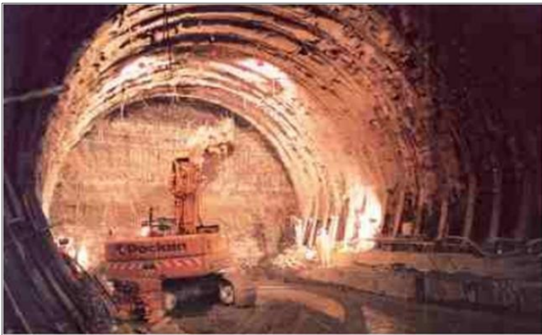
Figure II.11: Creusement à pleine section (BOUDJELLAL, 2020).
