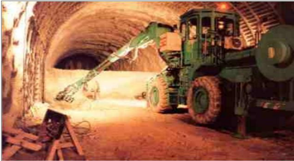
Figure II.12: Creusement en demi-section (BOUDJELLAL, 2020).
