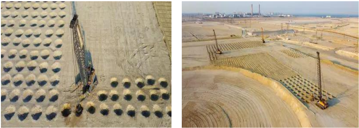
Figure II.10 : Chantier de compactage dynamique du sol ( https://www.bauer.de/en/soil-compaction-desert-kuwait )
