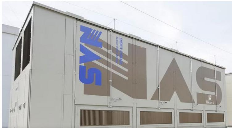
**Figure III.11.**Sodium-Sulfur Battery [189].
