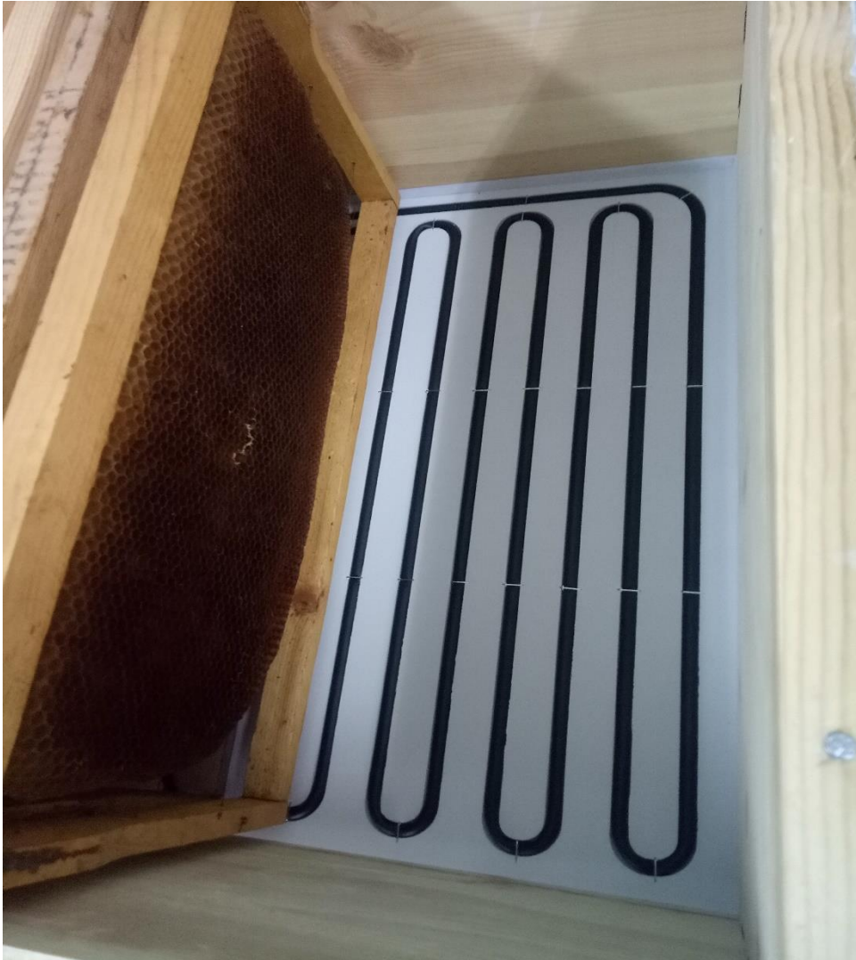
Figure 23. beehive after the Central Heater installation.
