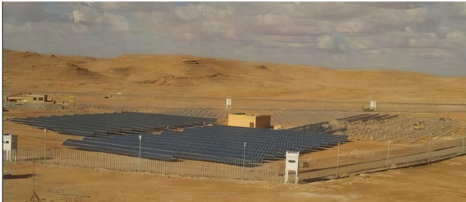
Figure III.4: Centrale PV Oude Nechou.
