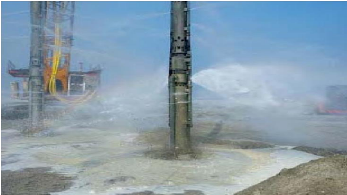
Figure II.3 : Vibro-compactage (Lawton, 2004).
