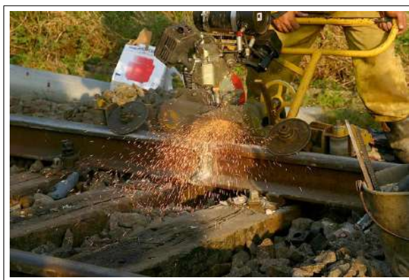
Figure 7.14. Meulage du rail.
