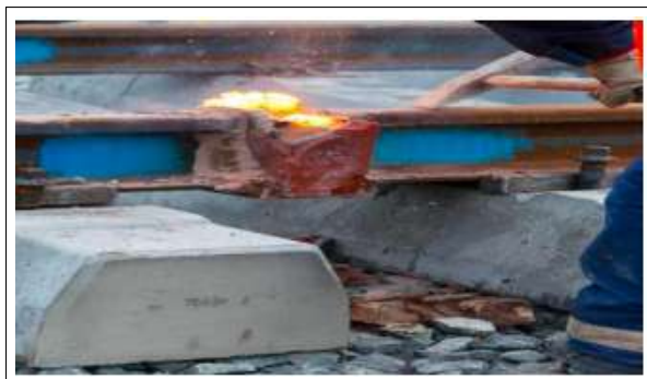
Figure 7.13. Tranchage du rail.
