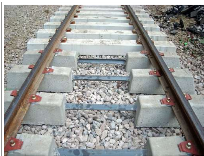
Figure 7.18. Traverse bi-bloc.
