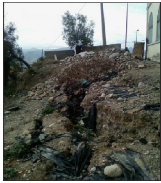
Figure 1.27: Photo montrant les fissures de traction.
