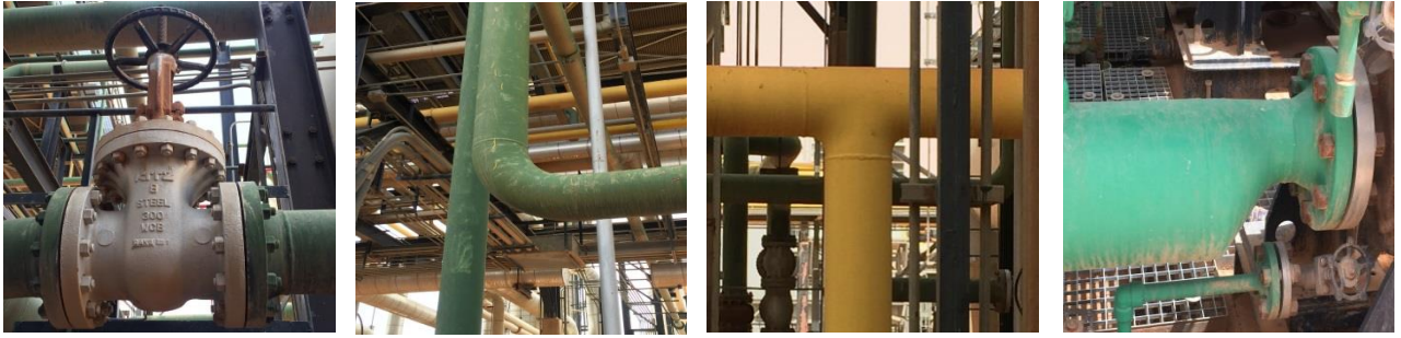
Figure I. 7 : Types de Raccords SONATRACH DP. Module 1, Hassi R'mel.
