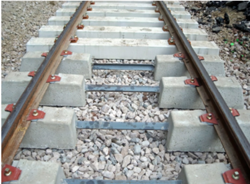
Figure VII.5. -Traverse bi-bloc
