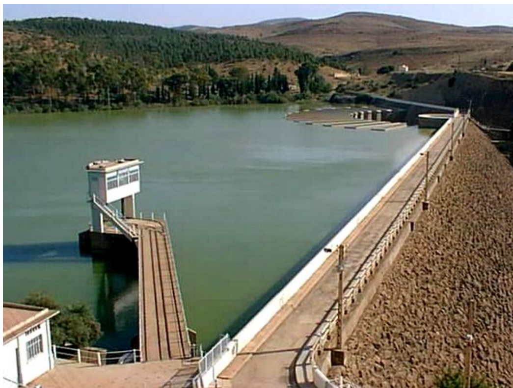
Figure VI.2: Digue du barrage BAKHADDA
