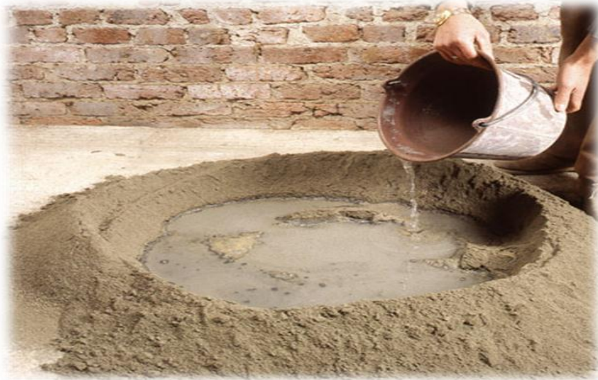
Figure 1.4 Eau de gâchage.
