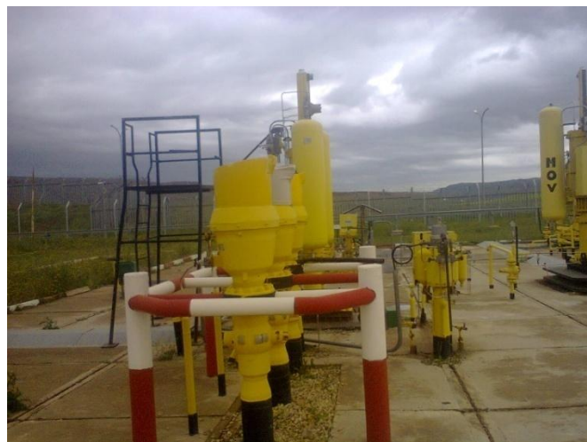
Figure 2 : Vanne By-Pass de la station SC4 Nador.
