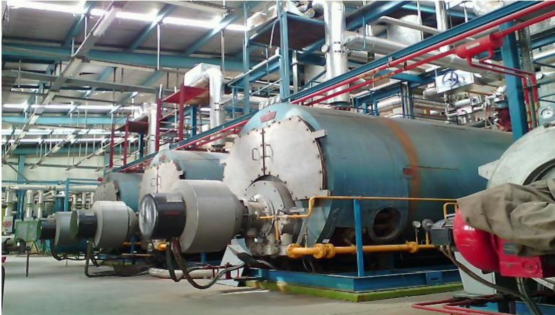
**figure-2.1-** chaudière \* type standard Kessel Duisburg
