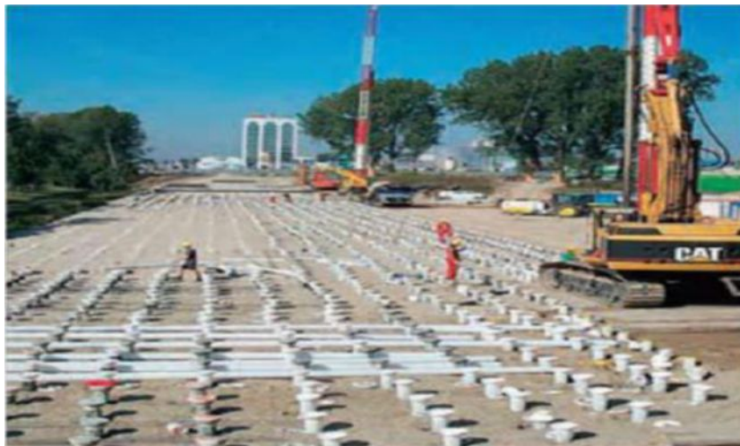
Figure II.4: Installation des drains.
