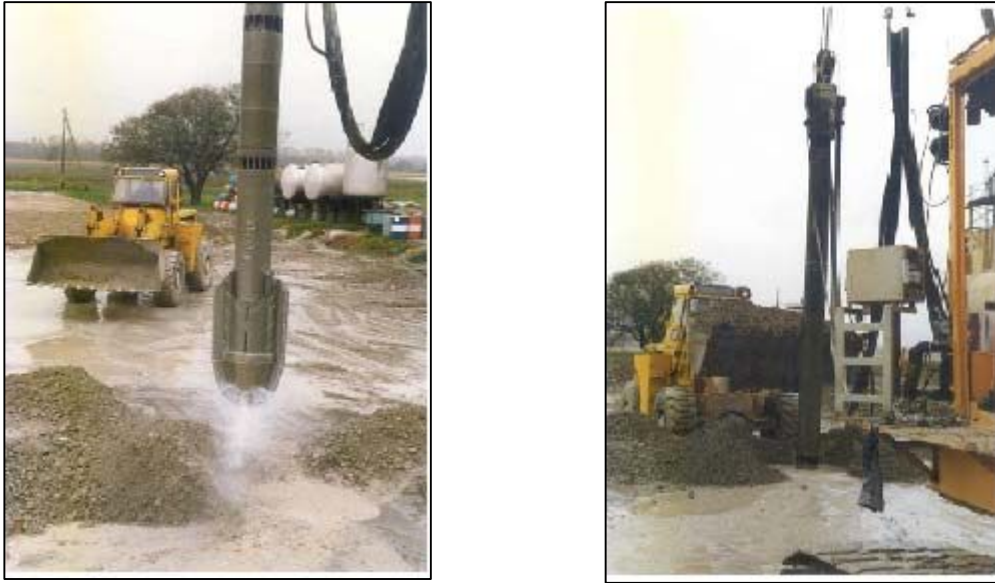
Figure II.30: Technique du vibroflotation
