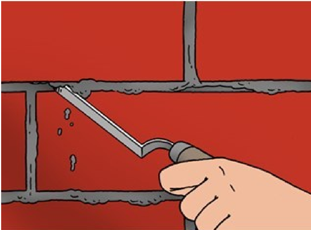
Figure I-05 : grattage des joints
